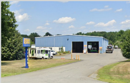
LEASE 1200 Route 9, Schodack 14,000 SF August 2024 HERC Rentals
