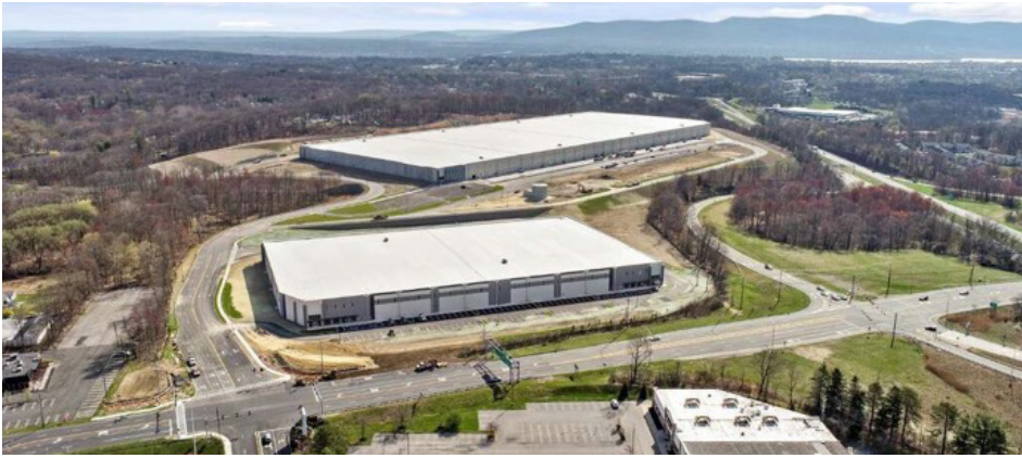
Newburgh Logistics Center
